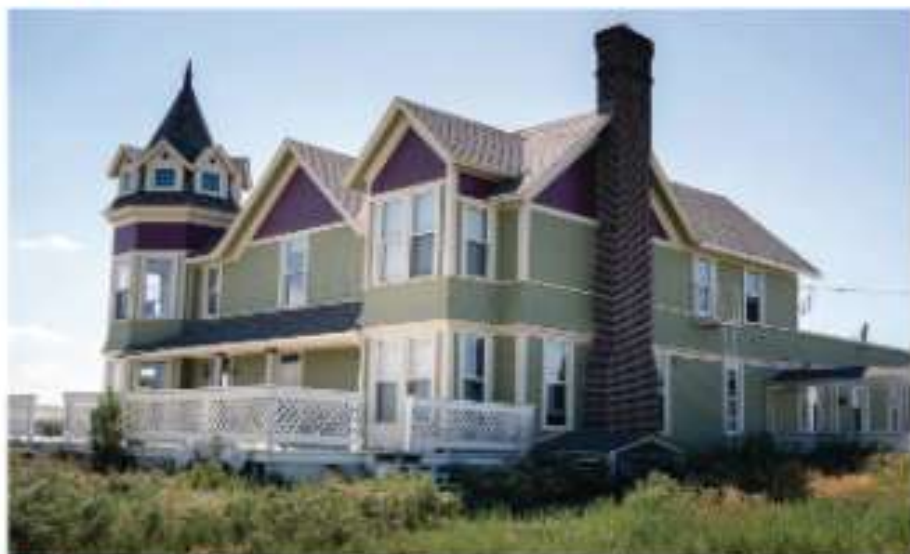
▲ Finished project, with historic colors, eroded over 40 years of neglect.
